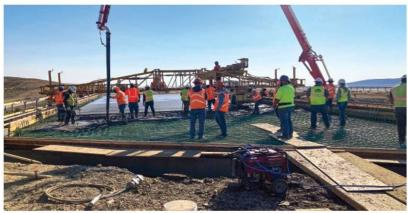
A crew with IHC Scott work on pouring concrete for a bridge deck at the Baxter Interchange on I-80 east of Rock Springs. The contractor and WYDOT were awarded an Excellence in Concrete Paving award this year by the Colorado/Wyoming chapter of the American Concrete Paving Association
